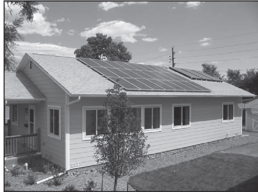
Figure 2. Twelve months of monitoring data confirm that the Habitat for Humanity house in Wheat Ridge, Colorado, is the first zero-energy home in the US. [Photo credit: National Renewable Energy Laboratory]
